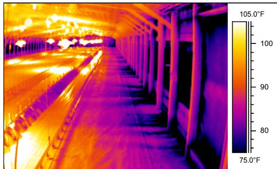
Figure 10. Cold air leakage.
