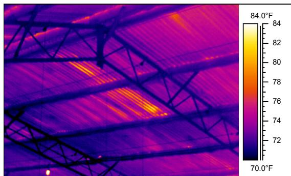
Figure 7. Ceiling insulated with spray polyurethane.
