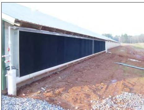
Figure 21. Poultry house evaporative cooling pad.
